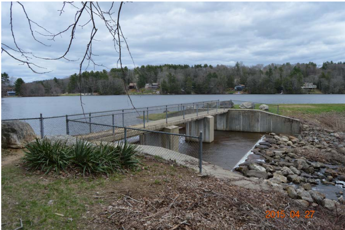
Photo 5a – Looking easterly from the right abutment toward the spillway and the beginning of a long earth embankment section that turns abruptly toward the right after the spillway.
