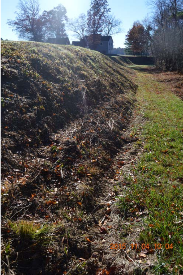
Photo 21n – An area showing what appears to be damage from mowing, as shown by the wheel ruts along the base of a steep slope section. Such areas could become susceptible to sloughing if not properly maintained.
