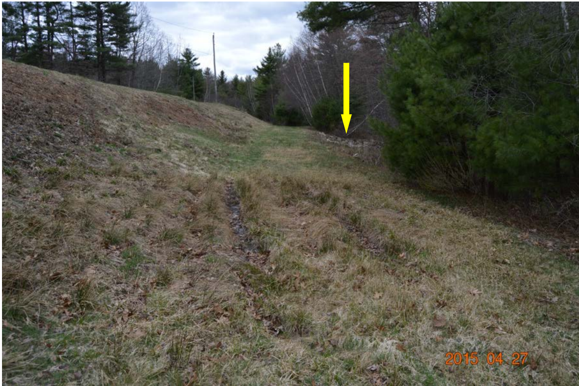
Photo 7c – A continuation of the downstream embankment slope and shelf taken from the sharp corner pointed out in the previous photo. The arrow points to riprap marking the discharge of the low level outlet passing through the dam.
