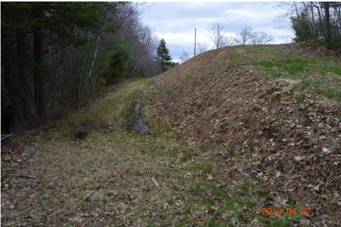
Photo 21g – This wet and rutted area is just beyond that shown in the previous photo, close to the left end of the main embankment.
