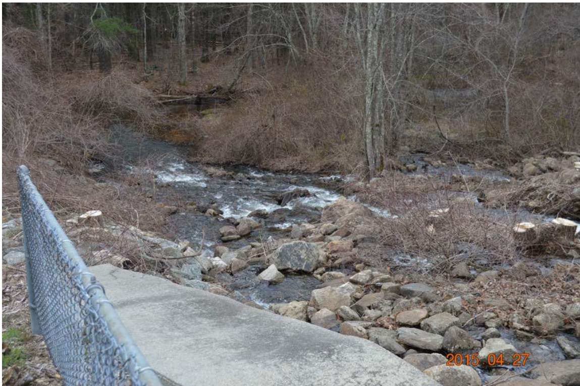
Photo 21c - Several large trees had been removed from the stilling basin area prior to a full inspection of the site, as evidenced by the stumps noted in this photo. Again, this area should continue to be monitored and brush removed on a regular basis.
