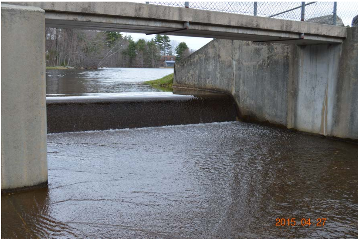
Photo 12a – An overview of the upstream portion of the left training wall
