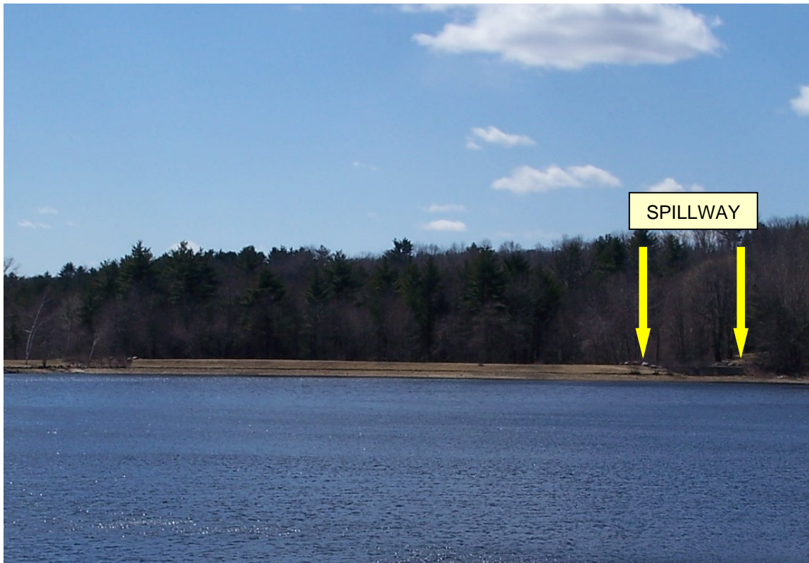
Photo 1 – The dam at Witches Woods Lake as seen from the upstream, looking south. The spillway, with extents shown by the yellow arrows, is situated directly adjacent to the right abutment of the dam. The dam itself, an earth embankment dam, extends out beyond the left side of the photo.
