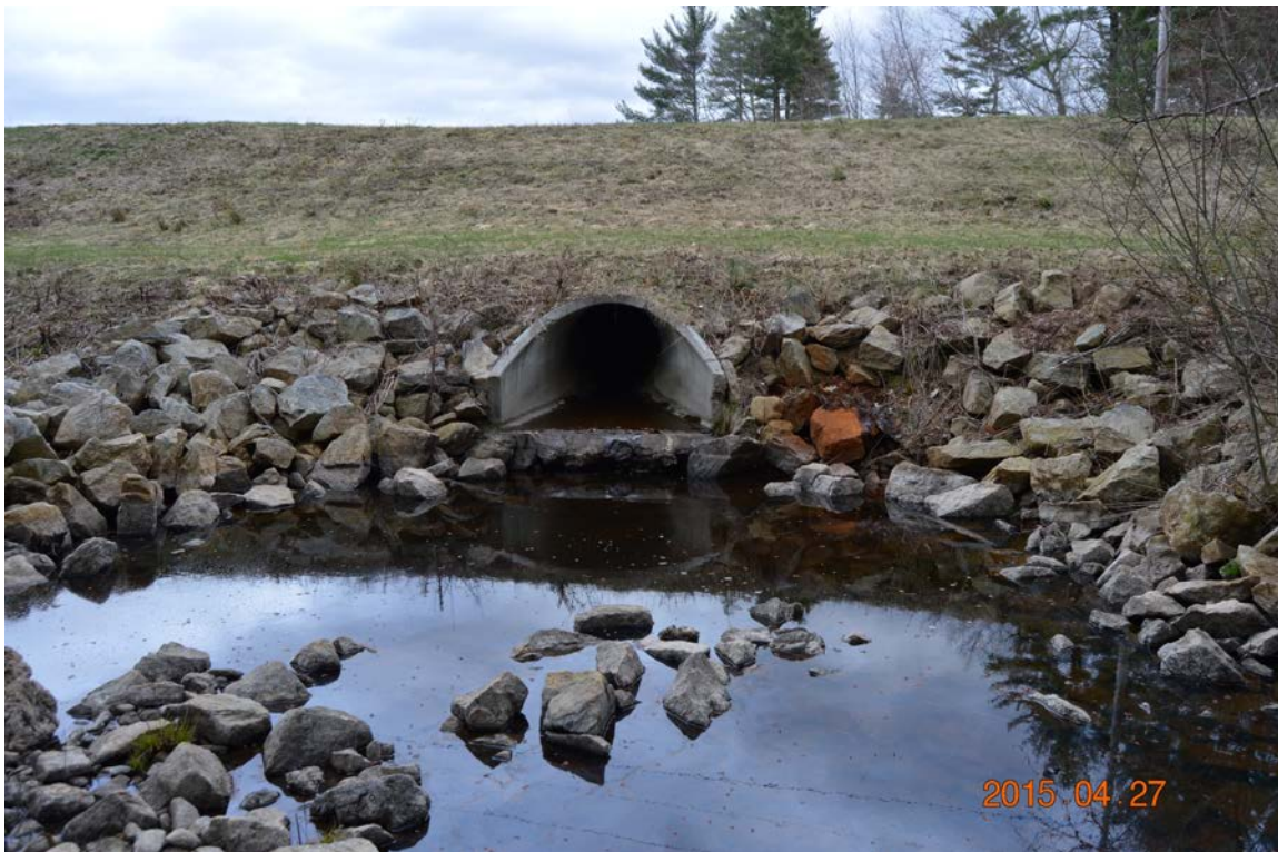
Photo 19b – A view looking upstream at the flared end pipe discharge point for the low level outlet pipe. There is no formal inlet point other than the structure previously shown at the water's edge in Photo 16.
