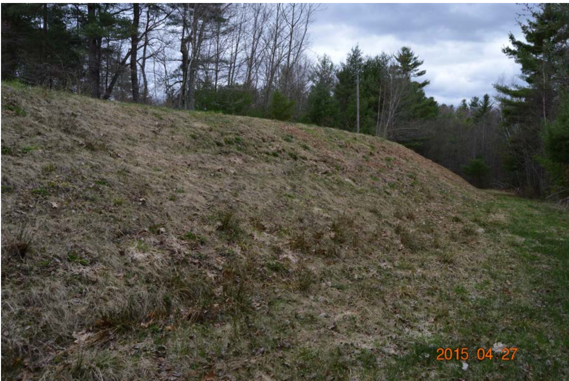
Photo 21m – A small area along the left section of the main embankment in the vicinity of the low level outlet area showing signs of what appears to be minor sloughing.
