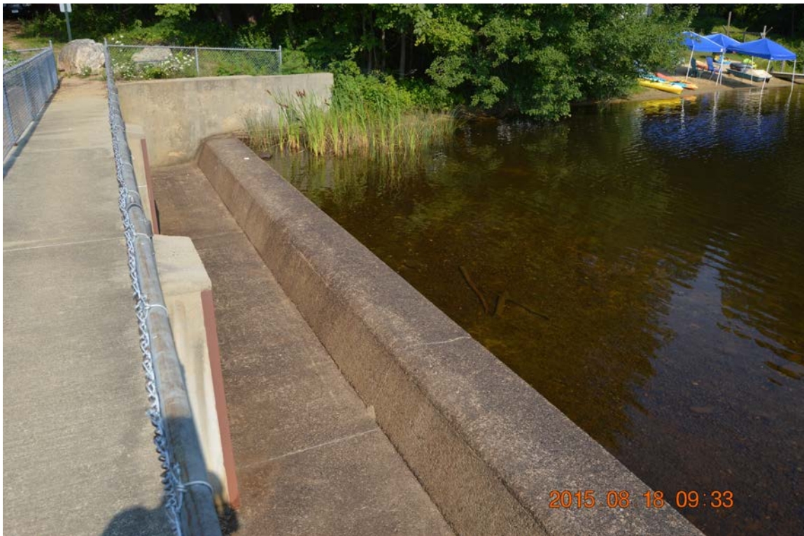
Photo 13b – The weir as seen from its left side during a low water level period. There are two control joints along its length.
