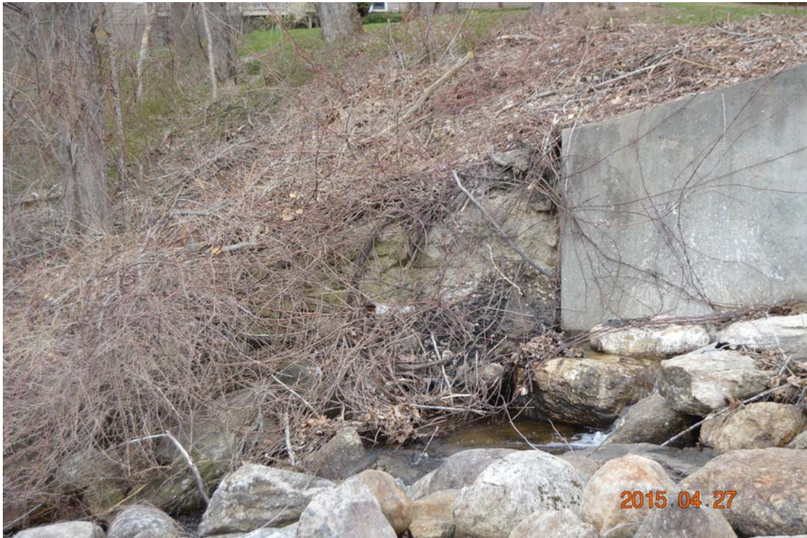
Photo 21b – The same situation with respect to susceptibility for dense growth along open riprap and side slope areas.
