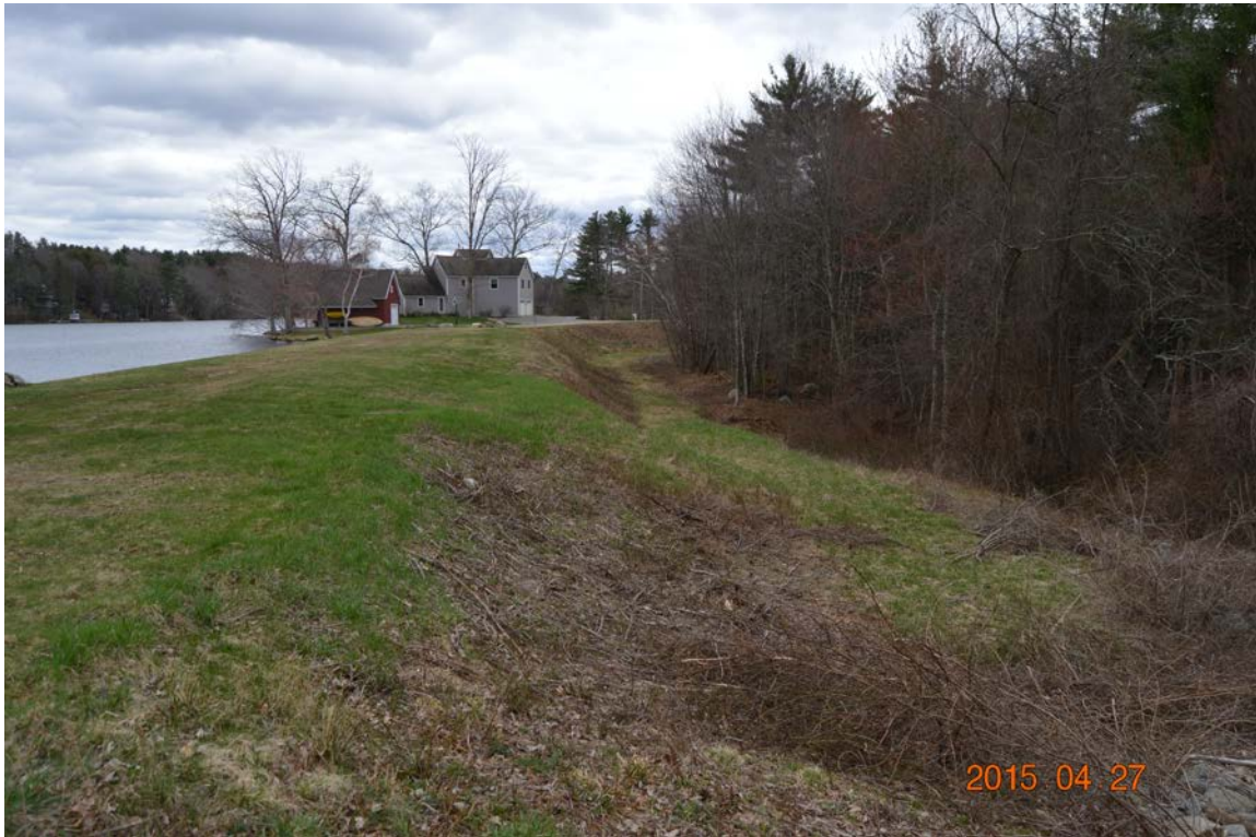
Photo 7a – The downstream face of the main embankment as viewed from the left side of the spillway. Note that there is a shelf along the downstream base of the dam, the height of which varies but has an average drop of about 2 feet across the length of the dam.
