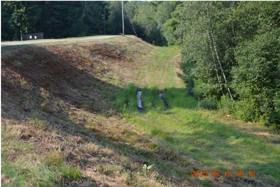
Photo 21h – The same wet and rutted area as shown in Photo 21e, but at a later date and a lower water level. Note that these wet areas persisted even with changes in water levels within the lake.
