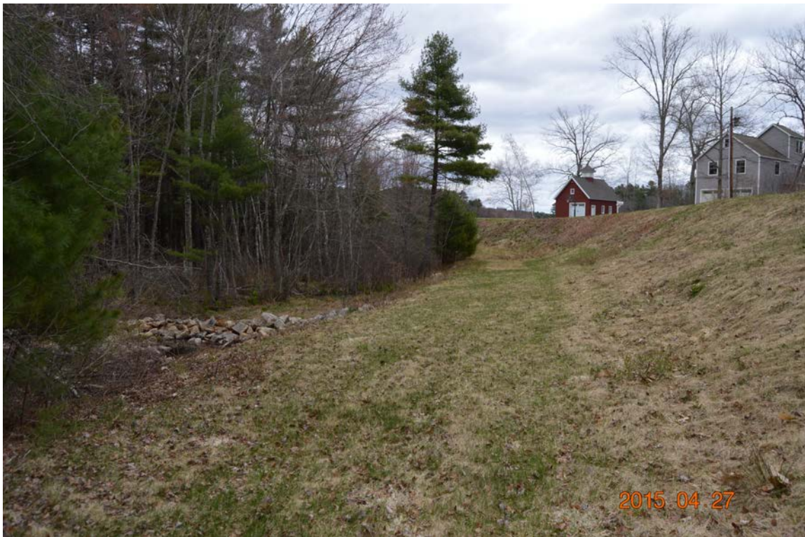
Photo 8a – The downstream face of the embankment as seen from the left abutment area of the dam. The riprap at the left center of the photo represents the discharge point of the low level outlet of the dam. The following photo will show the continuation beyond the sharp curve to the left beyond the red garage.
