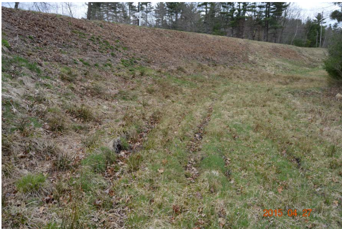
Photo 21d – A wet and rutted area near the right side of the sharp bend in the main embankment.
