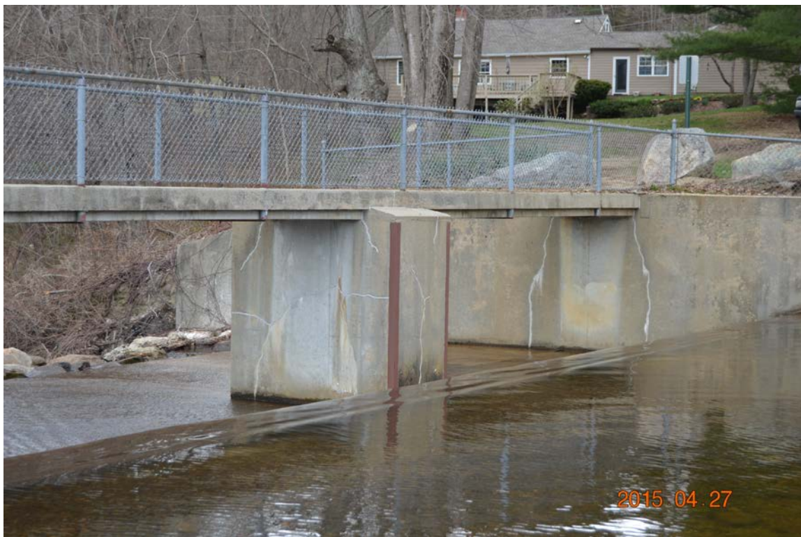
Photo 11a – The right training wall of the spillway as seen from the left upstream side. Note that crack lines along the faces of the walls and the bridge support piers, as seen in this and other photos of the spillway concrete surfaces, are actually filled with sealant. Cleaning and sealing of cracks along these surfaces was accomplished in 2012.
