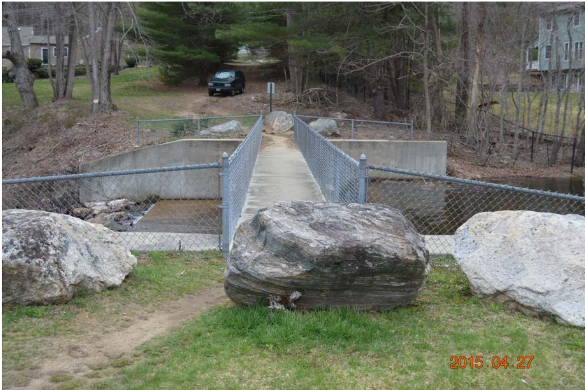
Photo 4c – Looking at the right abutment of the dam from the left side of the spillway. The dam ends directly after the spillway as the ground level rises sharply towards the west.
