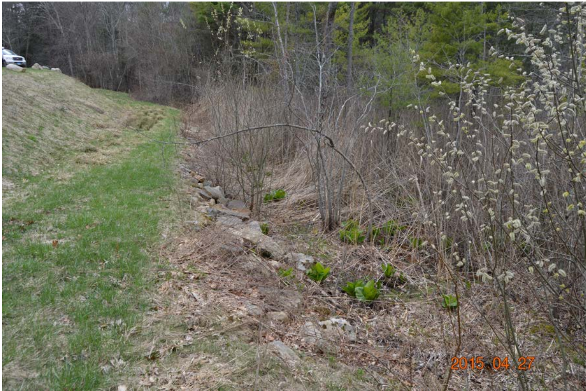
Photo 7e – The downstream embankment of the dike section, again with a base shelf between the toe of the dam and adjacent wetlands.
