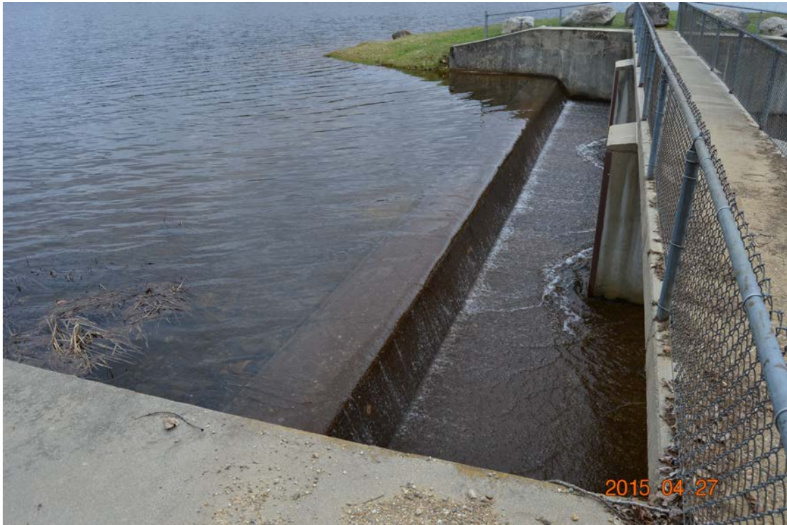
Photo 13a – The weir as seen from the right training wall area during an overflow period.
