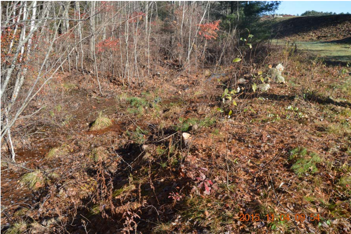
Photo 21j – An outlet from toe drains presumably installed or repaired in 1996, situated in the vicinity of the sharp downstream turn in the main embankment of the dam. Note the reddish stain indicative of a discharge characteristic of iron bacteria emerging from an anaerobic environment (e.g. within or below the embankment) to aerobic conditions, i.e., exposed surface water areas. Note also that in this area there is very little elevation difference between the downstream grass shelf and the adjacent wetlands.
