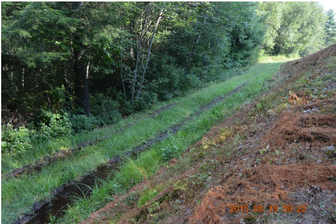
Photo 21i – The same wet and rutted areas noted in Photos 21f and 21g, this time tied together in a continuous stretch toward the left end of the main embankment. Note again the difference in saturation even with a lowered water level in the impoundment.
