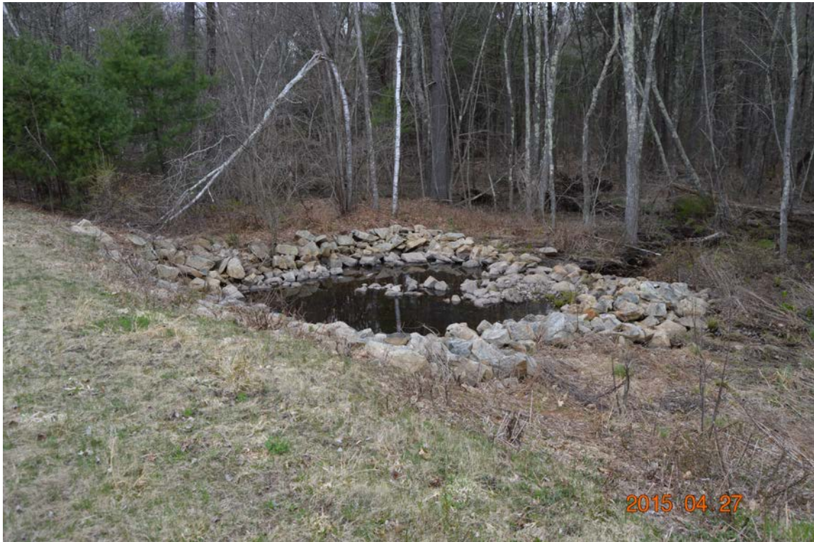
Photo 19a – The discharge area of the low level outlet pipe on the downstream side of the embankment. Note riprap protection to avoid scour.
