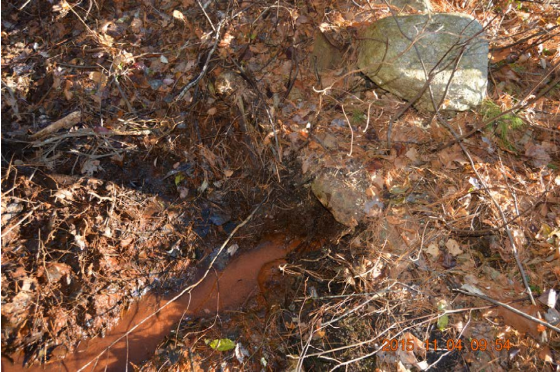
Photo 21l – Another toe drain discharge just north of the one shown in the previous photo, but without a visible pipe outlet.
