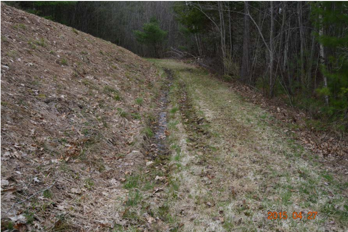
Photo 21f - A wet and rutted area near the left downstream end of the main embankment and just beyond the discharge point of the low level outlet.
