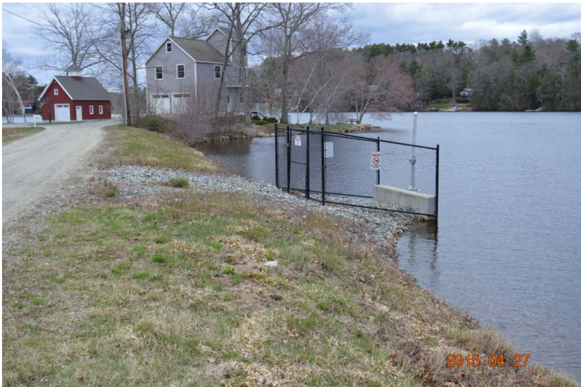
Photo 16 – An overview of the sluice gate structure on the upstream side of the main dam embankment. It consists of a sluice gate set along the vertical upstream side of a concrete wall.
