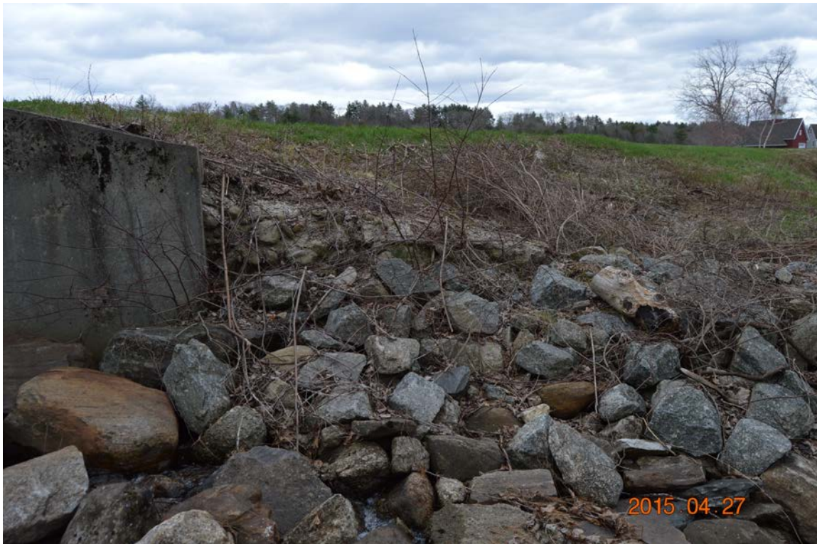
Photo 21a – The open riprap along the stilling basin area of the spillway creates an environment predisposed to the growth of dense brush and small tree growth within its open joints. Although tedious, these areas should be monitored and kept clear of such growth. This view looks toward the end of the left downstream spillway training wall.
