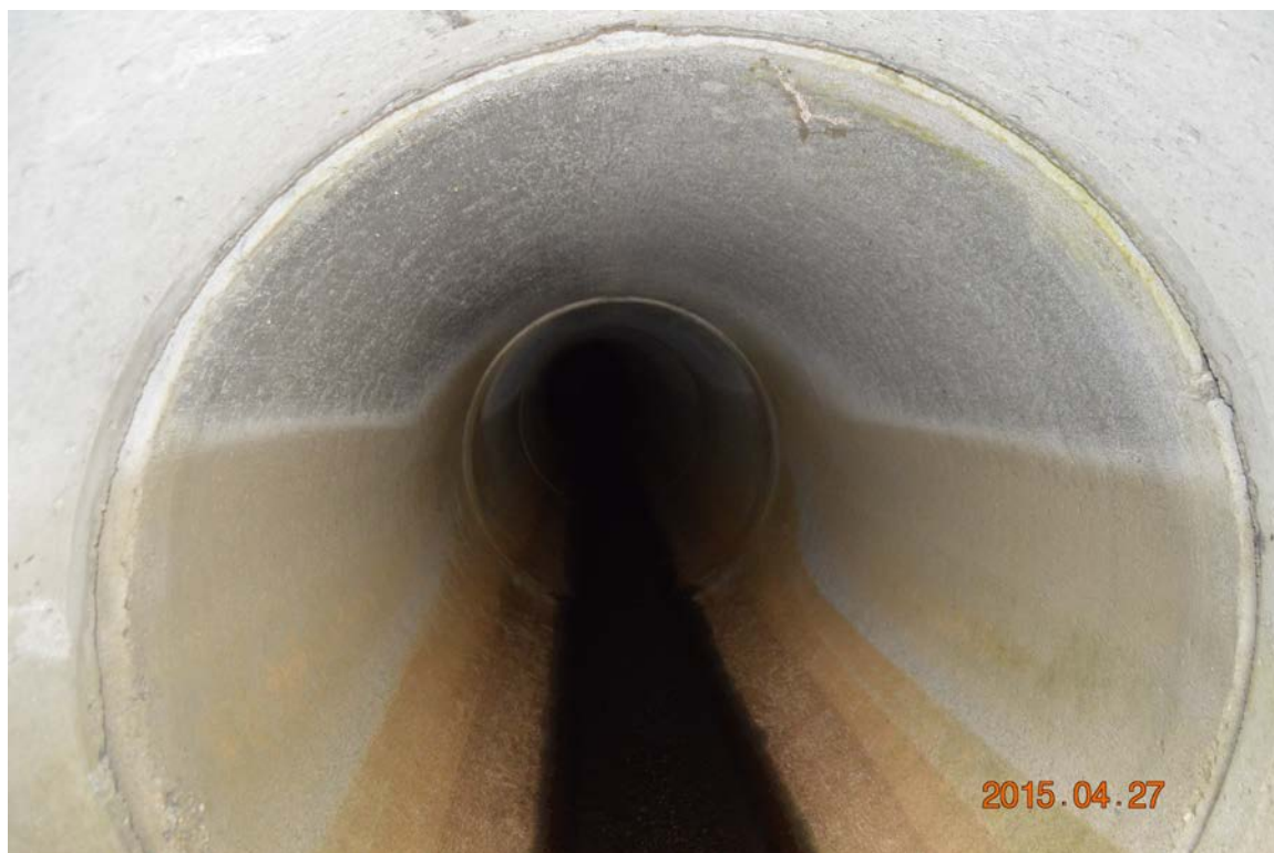
Photo 17 – Since there is no gatehouse interior, we have chosen to show the interior of the low level outlet pipe, which is in good condition with no structural issues and no apparent open joints.
