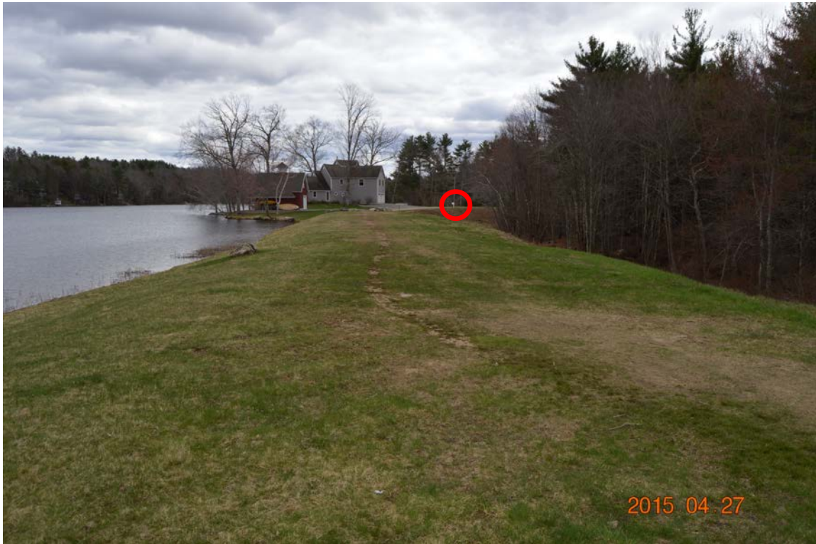
Photo 5b – The crest of the dam looking southeasterly towards a sharp bend (to the right) in the embankment at the house location. The spillway is just behind and outside the viewpoint of the photo (see prior photo). The next photo shows the crest area just beyond the house in the distance, at which point the dam embankment takes a sharp turn to the right.
